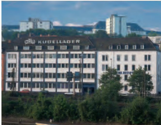
Administration and production facilities in Würzburg
